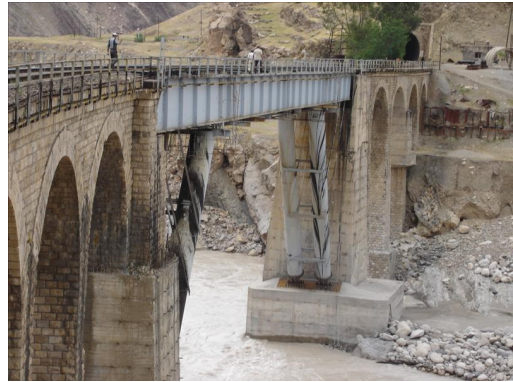
Fig. 2. Shazand bridge after two retrofitting
