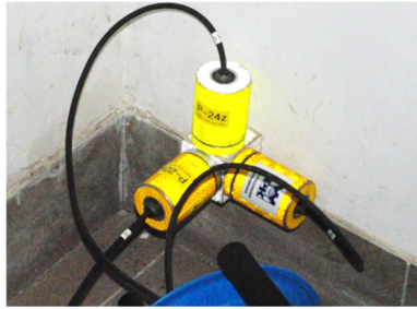
Fig. 3. Acceleration sensors mounted on the foundation of the building
