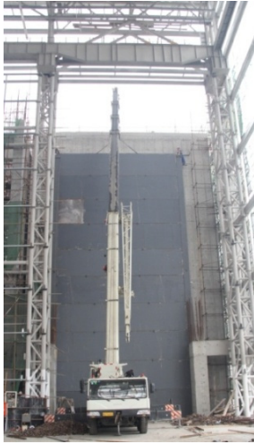
Fig. 5. Construction photo of the door
