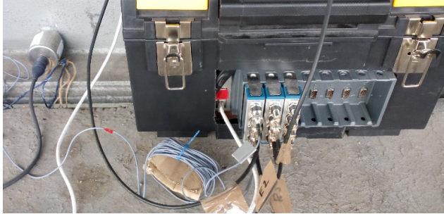
Fig. 3. The cRIO 9074 with three NI 9234 modules connected via Wi-Fi antenna
