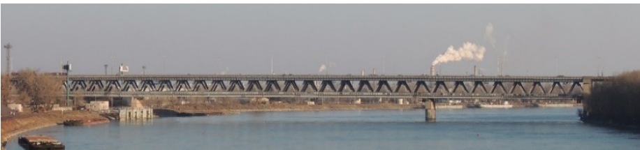
Fig. 2. The multi-span truss bridge (Bridge No. 2)
