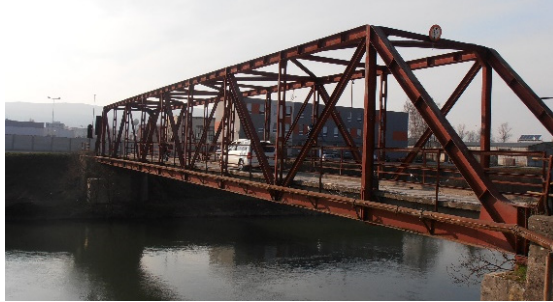
Fig. 1. The single span truss bridge (Bridge No. 1)
