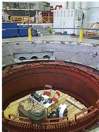
Fig. 1. View of the generator stator in a repairing phase
