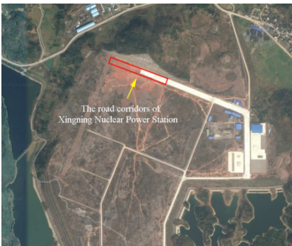
Fig. 4. The overview of the Xianning Nuclear Power Station
