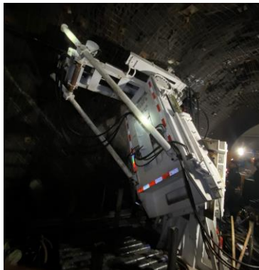
Fig. 6. Construction state in coal mine
