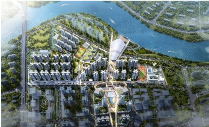
Fig. 1. Typical metro depot superstructures
