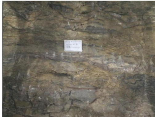
Fig. 2. Typical surrounding rock of tunnel face (Photographed by Rui Qu, Jiedexiu tunnel, 2016)
