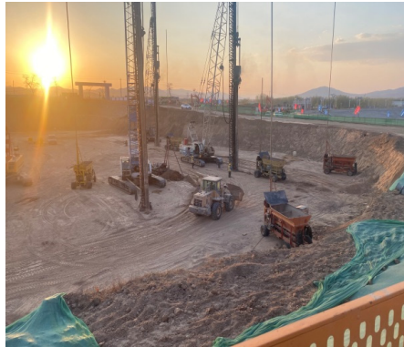
Fig. 1. Test site of lime soil compaction pile
