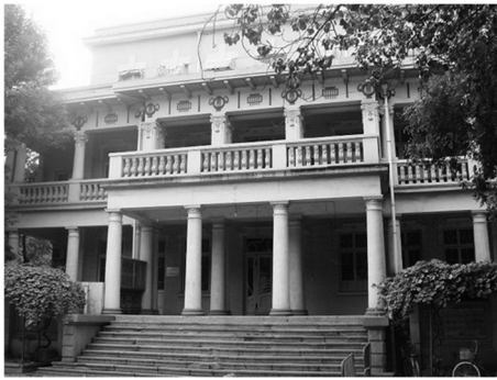
a) Architectural appearance of building A
