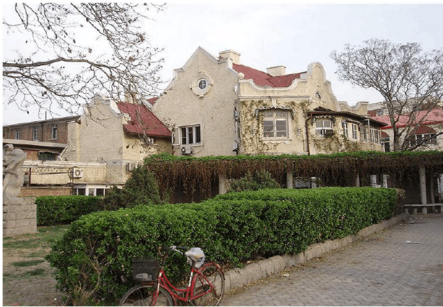
a) Architectural appearance of building C
