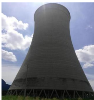
Fig. 3. Double curve cooling tower to be dismantled
