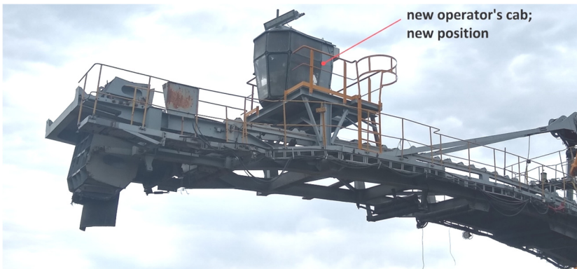
Fig. 8. New cabin layout on the bucket wheel excavator's landing belt SRs400.14/1
