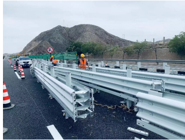
Fig. 23. Photo for guardrail installation at construction sites
