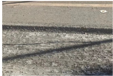
b) Road surface after milling
