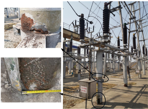
Fig. 1. Zhenyang 220kV substation's corroded steel columns
