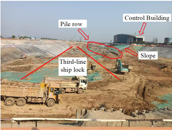
Fig. 13. The layout of pile-anchor support section for the third-line ship lock. Photo taken by Yuchen Liu at the Caijiashou project site in Wangcheng District, Changsha City, Hunan Province on January 2024
