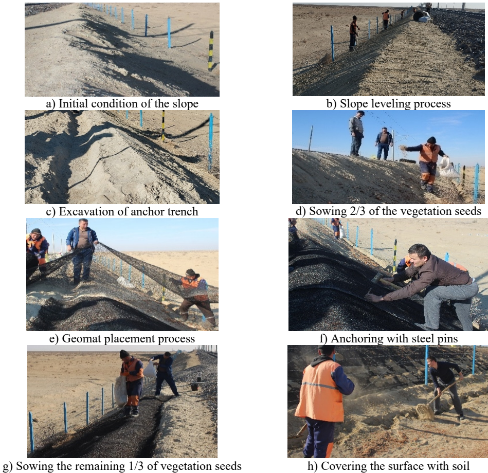
Fig. 2. Installation of Geomats on the Slope at Qorlitog'-Kiyikli Section. Photos were taken by the article's author A. Sh. Uralov during field research on the Bukhara-Miskin railway line (Qorlitog'-Kiyikli section) in November 2024
