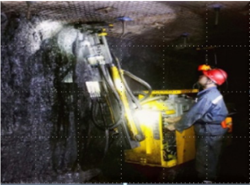
Fig. 5. Installation of anchor rods and sensors
