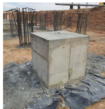
Fig. 1. The location of the pile in the building plan under number 13, whose load-bearing capacity has been established. Photo taken by the author at the Tebinbulok site on November 1, 2023 Fig. 2. A concrete cube for the test pile's hydraulic jack placement. Photo taken by the author at the Tebinbulok site on November 13, 2023
