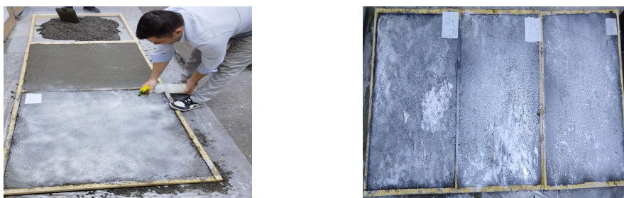
Fig. 2. Application of film-forming materials to the surface of freshly laid cement concrete. Photograph taken by Tukhtayev Matchon Bekjonovich in the laboratory and on field test sections of newly constructed cement concrete pavement, Tashkent, Uzbekistan
