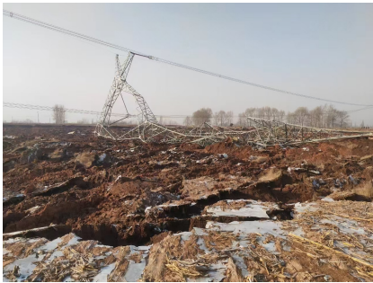
b) After the site liquefaction in Caotan Village. Team member Cheng Zhenglun took this photo in Caotan Village, Qinghai Province, China on December 9, 2023
