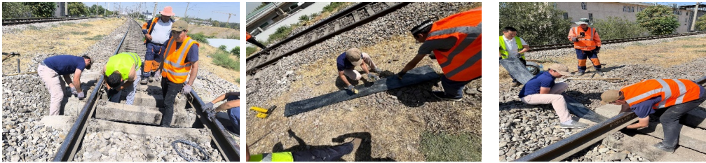
Fig. 3. The process of installing elastic sleeper pads in the rail joint zone. The photograph, taken by the third author on August 29, 2025, shows the process of conducting experimental research on the installation of elastic under-sleeper pads
