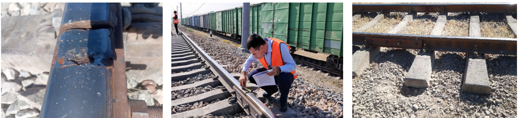
Fig. 1. Defects in the rail joint zones. The photograph, taken during research conducted by a third author in 2024-2025, depicts the process of studying issues in the railway superstructure elements within the rail joint zones
