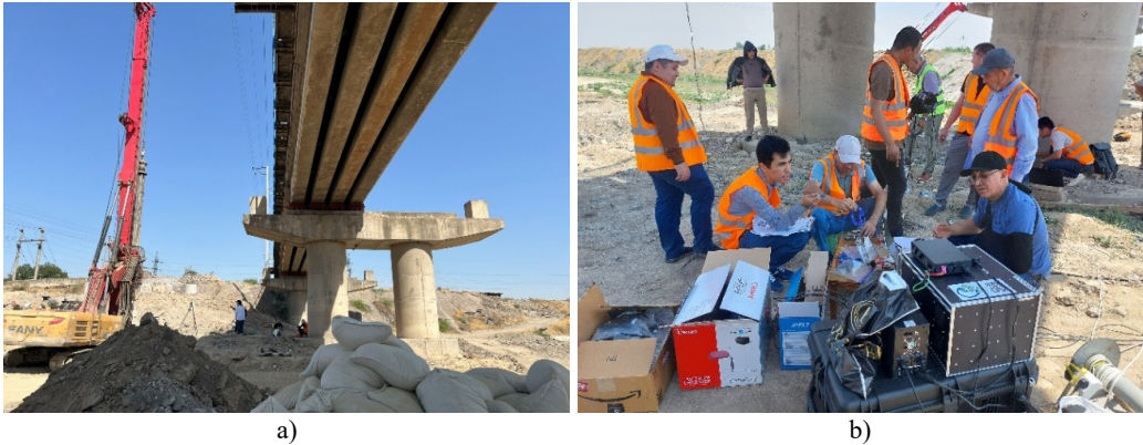
Fig. 1. Bridge's photo and photo of the monitoring studies in progress: a) photo of the bridge, b) photo of monitoring studies in progress. The photos were taken by S. Takhirov on May 30, 2025
