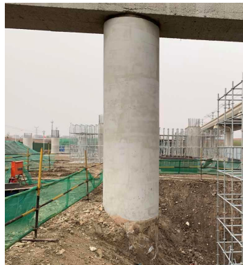
Fig. 12. Strengthening concrete pouring effect diagram (Construction site at Changchun, Jilin, China, 2023.5.10)
