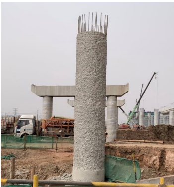
a) Roughening treatment of original pier concrete surface
