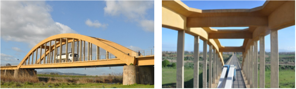
Fig. 3. Views of the arch stayed bridge 1 as second case study Photo by the authors during field investigation
