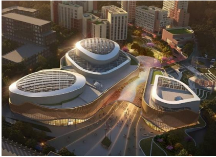
Fig. 2. Aerial view of the performance theater. Photo by Sun Dianlong, Shenzhen, China, Jan 24, 2024
