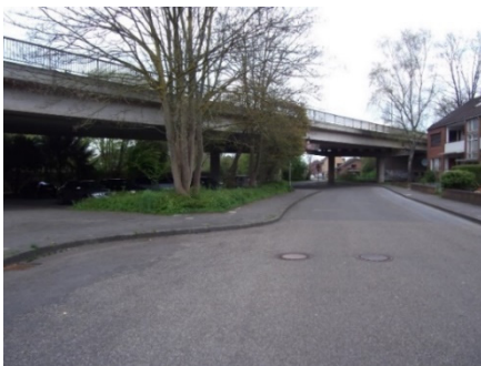
a) General view of the bridge
