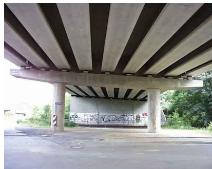
b) Underside view of the bridge
